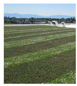
to be placed directly on top of almost any roofing membrane system, eliminating the need for additional drainage, filtration or root barriers.
